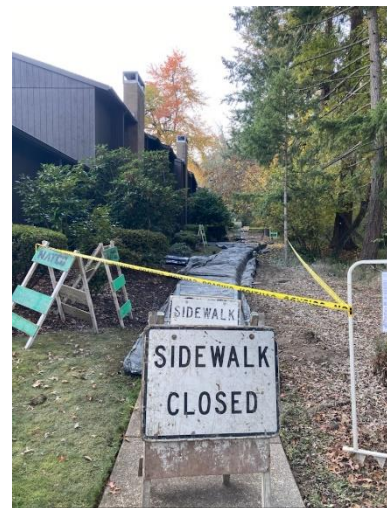
Sidewalk work 141 to 149 Westbrook Way
