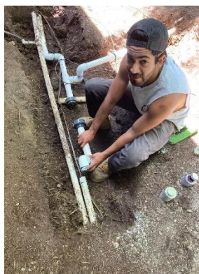
Repair of freeze damage in front of 135 Westbrook Way. Does it seem like it got that cold this winter? Contract laborer Zain.
