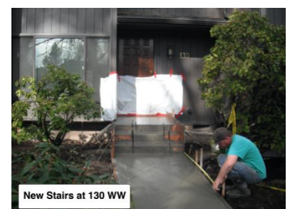
New stairs and sidewalk at 130 Westbrook Way
