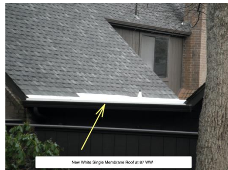
87 WW New Roof
