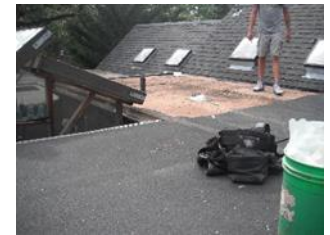
Roof Repair at 132 Brae Burn
