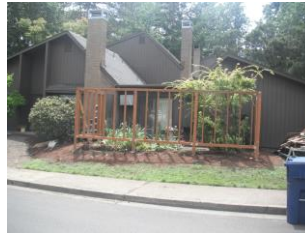
Patio Wall Repair at 10 Brae Burn
