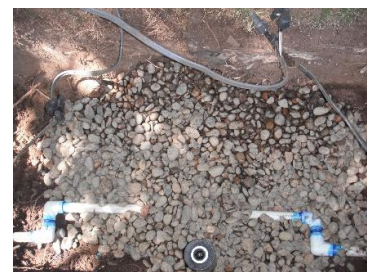
Irrigation and Electric Repair Driveway 4
